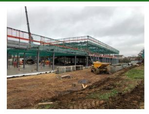
The main steel frame, floor planks and the first staircase have now all been completed. ISG are currently working on the lift pit and the second staircase. Scaffolds have been erected for access for the plank and roofing contractor; floor and nets for roofing and the steel framing system have started. The next phase will be to commence work on the roof.
